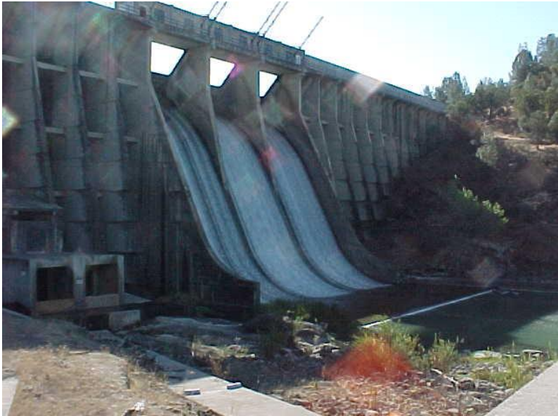
Stony Gorge Hydro Project
